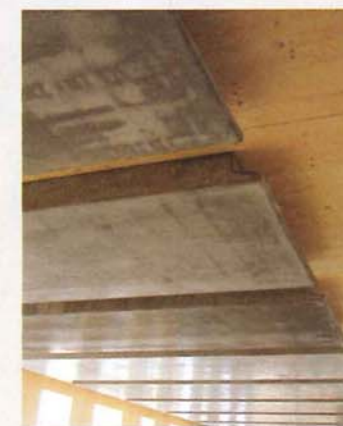
Concrete radiators installed.
