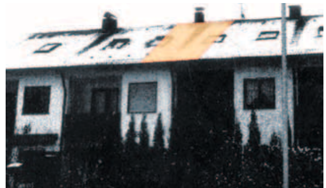
Fig. 5: The same amount of heat is lost per metre of a thermal bridge at the top of the masonry as on three square metres of undisturbed roof area. Weaknesses in the roof area can be easily visually identified in this image from the melted snow.
