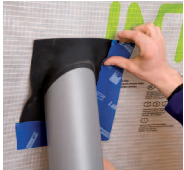
Fig. 11: If the penetrations cannot be avoided, suitable and approved systems should be used for sealing. A quick and permanently tight mounting will justify the additional costs [with the kind support of the company pro clima 2011].
