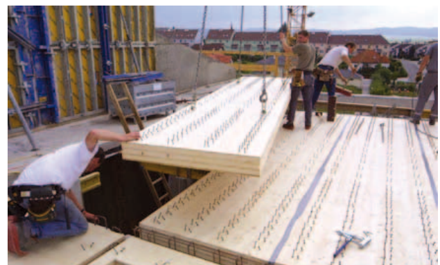
On site assembly of elements with screw connectors ( www.ancon.at )
