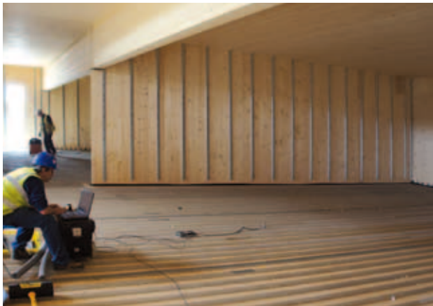
Preparation of KLH® TCC elements for pouring the concrete on site (TimCrete © Ramboll)
