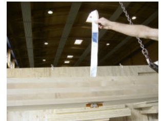
4. Lifting situation with built-in FB system
