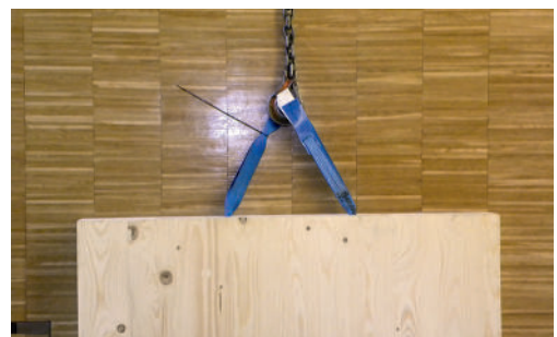
If the lifting gear is installed in pairs, the lifting hook must be hooked into both loops
