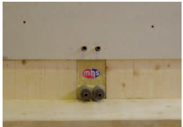
Facing of KLH® solid wood panel and Instabox – in this case with a type X gypsum board.
