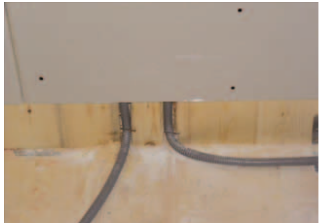
Fig. 67 – Electric cables in floor structure
