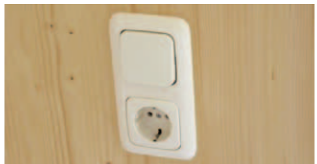
Fig. 54 – Installation of a switch/wall socket combination for walls with visible surfaces. The drill hole on the visible side must be sized according to the socket diameter and the covering frame (usually 68 mm diameter)
