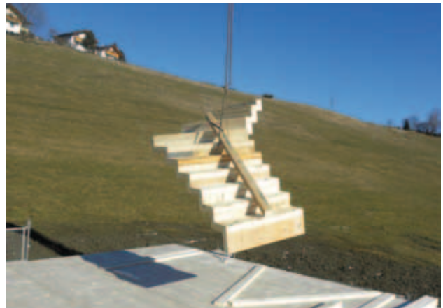
Fig. 48 – Assembly of a prefabricated flight of stairs
