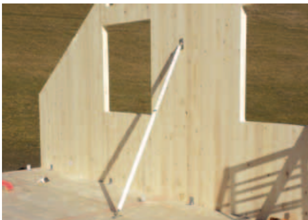
Figs. 43 to 46 – Assembly of KLH® components
