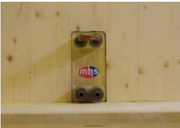
Installation of an Instabox for a valve radiator.
