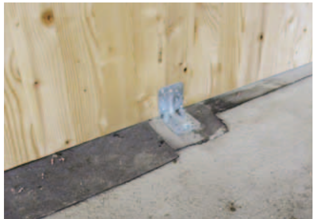
Fig. 38 – Moisture sealing
