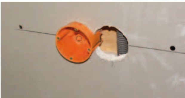
Fig. 52 – Installation of type X gypsum boards by a dry construction worker and socket drilling in the course of that process
