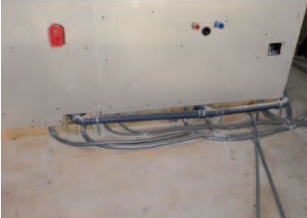
Fig. 64 – Connection of washing machine, washbasin
