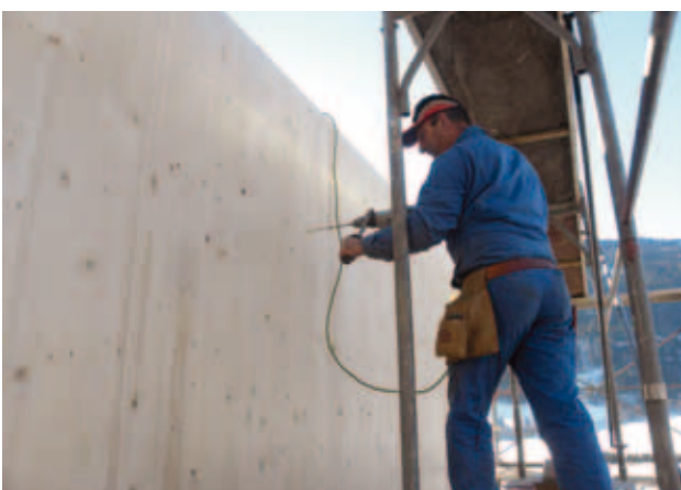
Figs. 39 to 42 – Assembly of KLH® components
