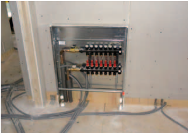
Fig. 66 – Floor distribution cabinet
