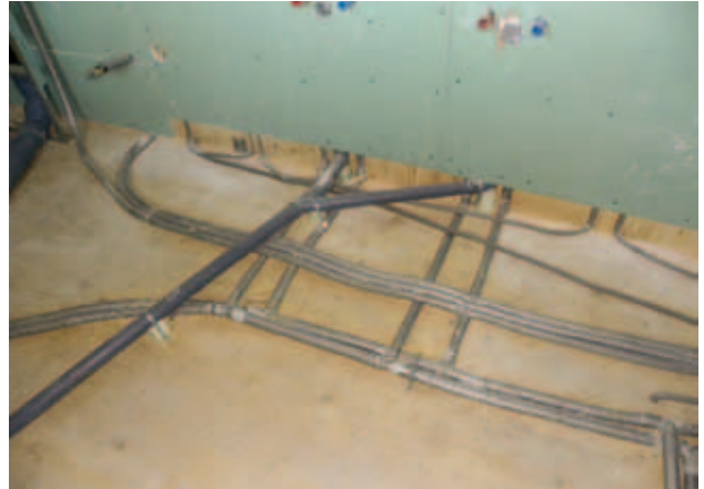
Fig. 65 – Connection of double washbasin
