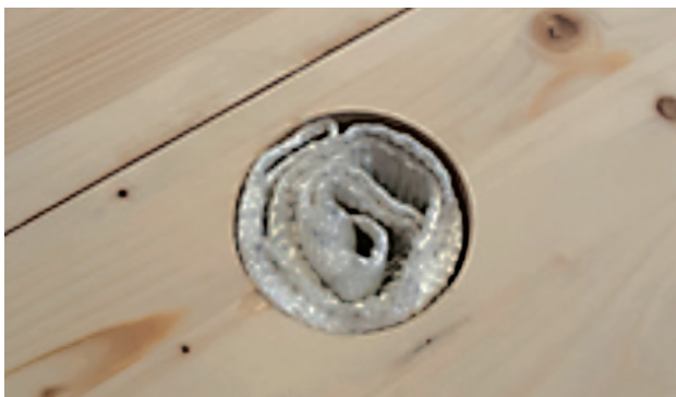
2. Transport situation with rolled-up loop in the blind hole
